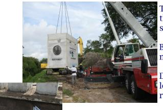
Technology is based on slowing the flow's velocity to facilitate settling.
