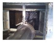
Servicing the EcoVault is easy with the accessible hatches and requires a vacuum truck.
